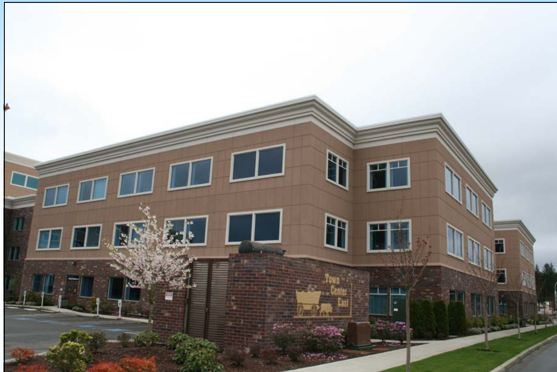
Tumwater Town Center is more than 250,000 sq. ft. of design-build work for Betschart Electric.
